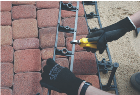
You can create a curved surface border by cutting the lower strip of the edging.
