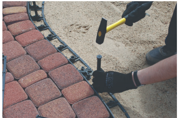
Garden Edge Pro borders are fixed to the ground with nails:
